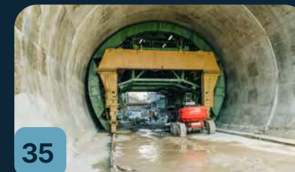
Scaffolding, shoring and formwork
